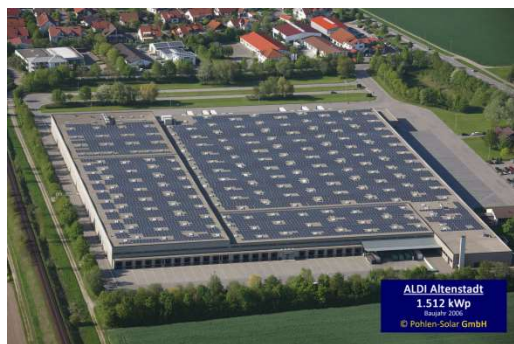
Figure 1: The PV power plant at the Altenstadt site in Bavaria has been in operation since 2006.
